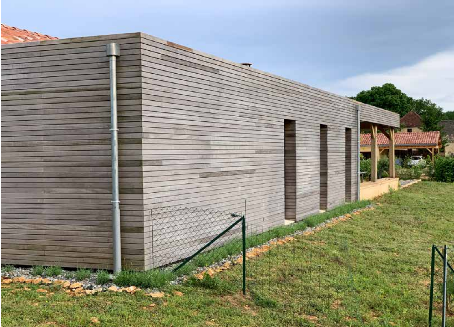
Project: Private House. Facade cladding in LDCwood® ThermoWood® ayous BELO profile. Planned by Lemahieu Group®.
